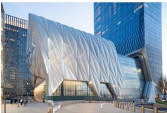
Movable Exterior Shell - The Shed Art Centre
